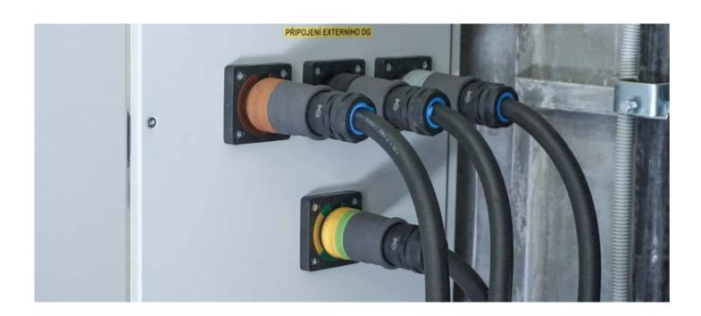
Having a single, standardized connector system for all power distribution equipment in the country saves crucial time in case of an emergency.
